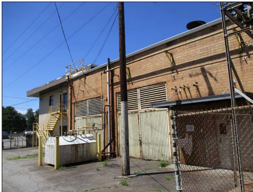
Photograph 30: View of east elevation of Catawba Complex; looking southwest. (2017)
