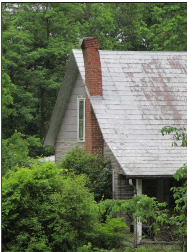
Photograph 5: Detail of northeast elevation of J.M. Orders House.; looking south. (2017)
