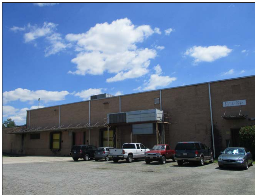
Photograph 25: View of addition on west elevation of Catawba Complex; looking northeast. (2017)
