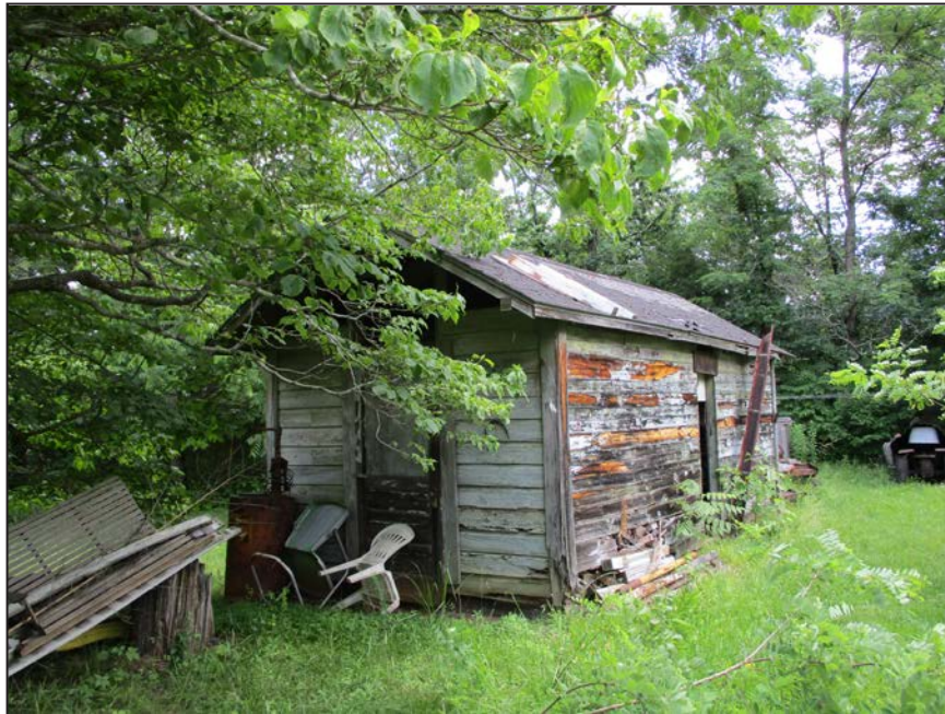
Photograph 10: Oblique view of Shed 1; looking east. (2017)
