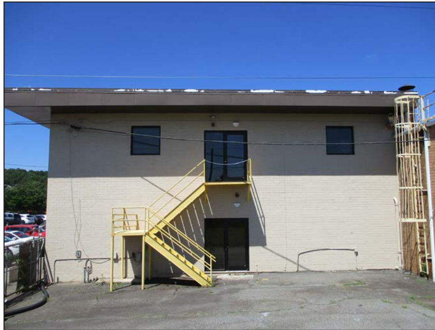
Photograph 18: East elevation of 2-story New Formalism addition of Catawba Complex.; looking west. (2017)
