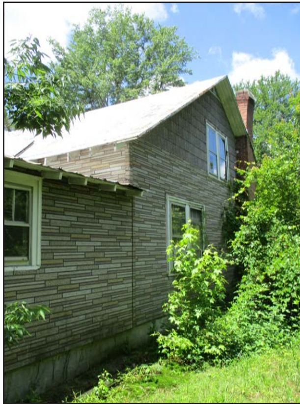
Photograph 6: Detail of northeast elevation of J.M. Orders House.; looking west. (2017)
