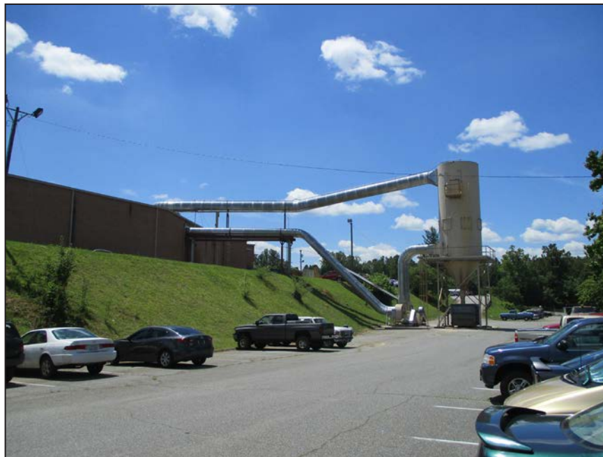
Photograph 22: Oblique view of of Catawba Complex and non-contributing silo; looking southeast. (2017)
