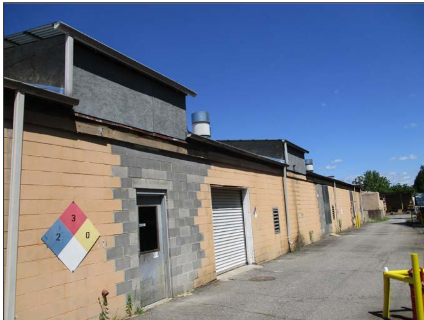
Photograph 32: View of east elevation of Catawba Complex; looking northwest. (2017)
