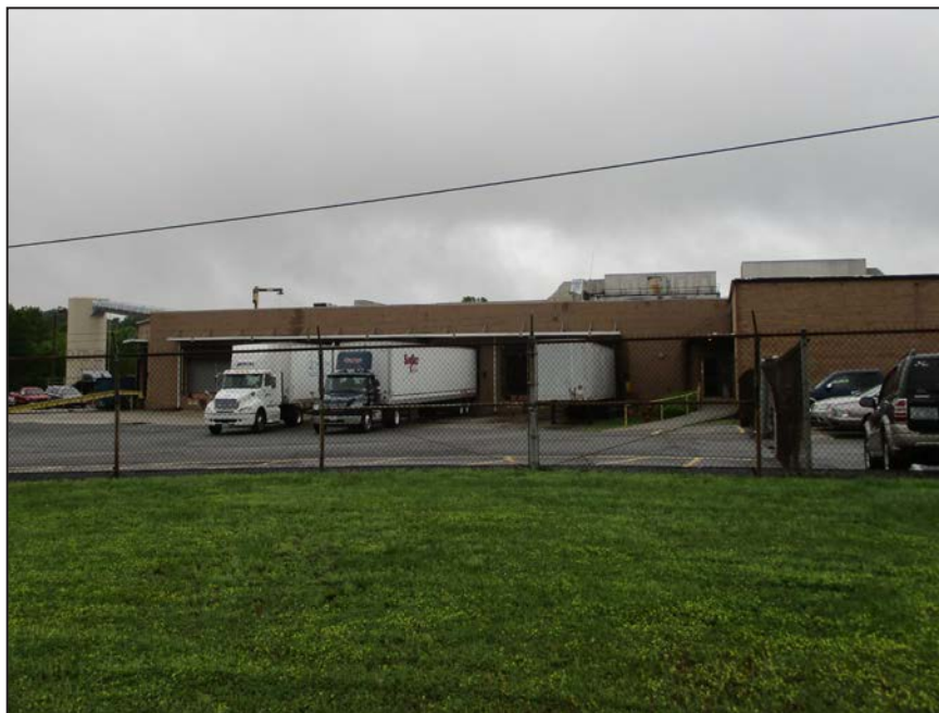
Photograph 19: View of loading dock on façade of Catawba Complex; looking north. (2017)
