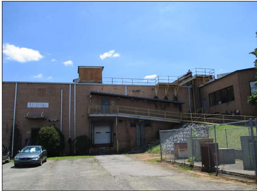
Photograph 24: View of west elevation of Catawba Complex; looking east. (2017)
