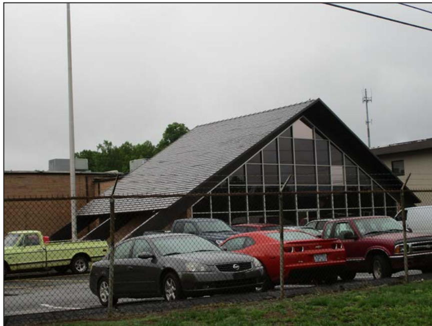
Photograph 16: Detail of A-Frame entrance bay of Catawba Complex; looking northeast. (2017)
