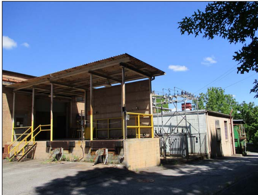
Photograph 36: View of loading dock, electrical substation, and concrete block addition on east elevation of Catawba Complex; looking northwest. (2017)
