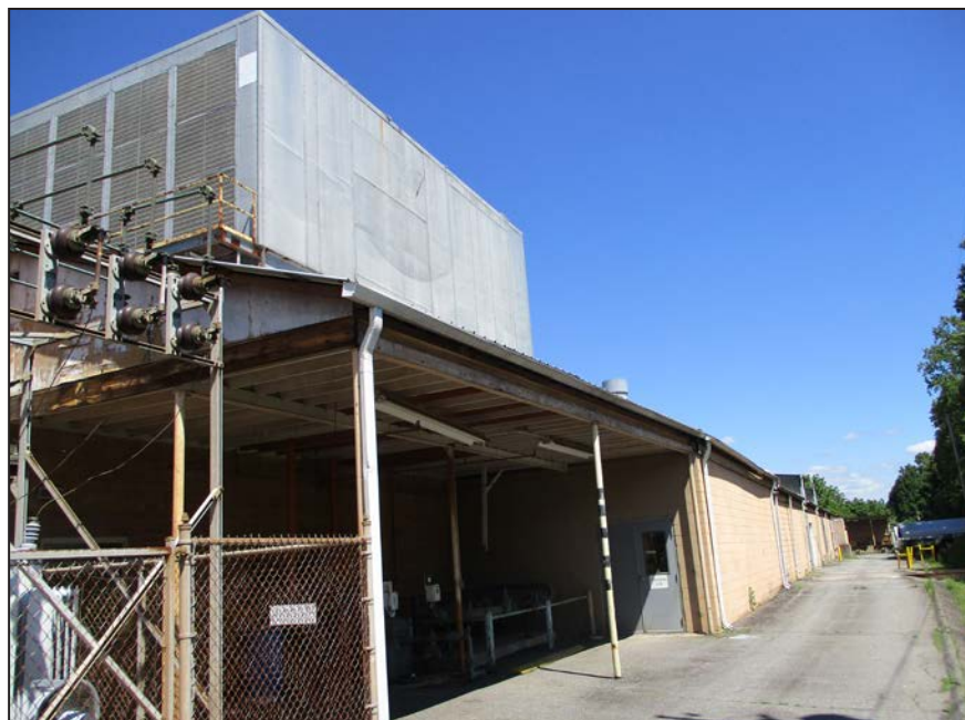
Photograph 31: View of east elevation of Catawba Complex; looking northwest. (2017)
