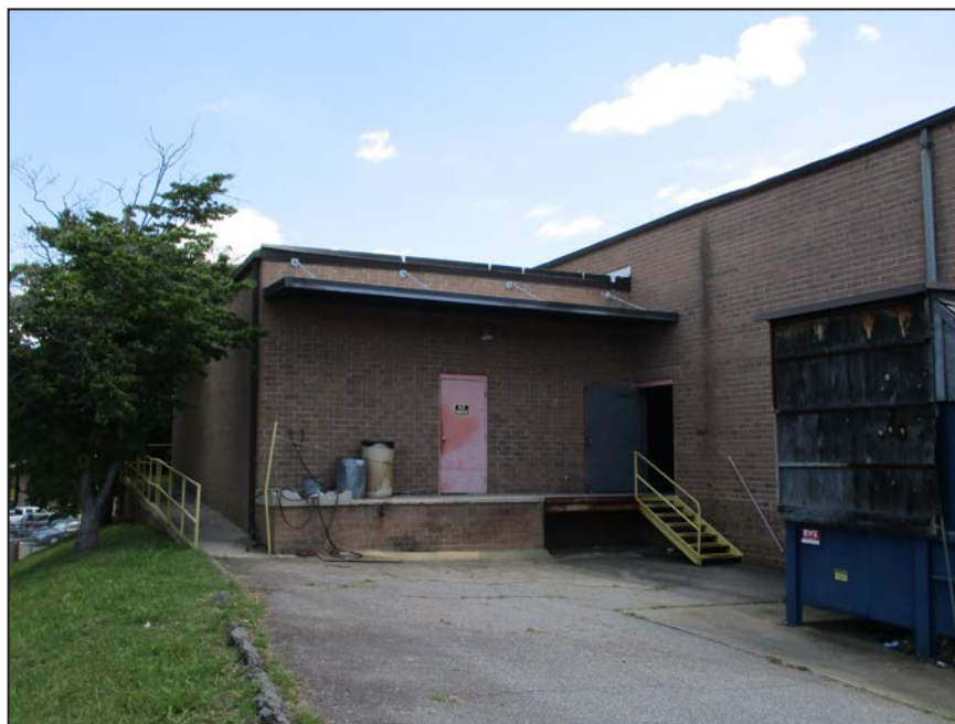
Photograph 23: View of addition on west elevation of Catawba Complex; looking northeast. (2017)
