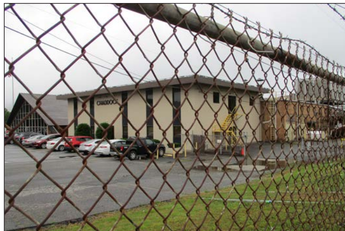
Photograph 14: Oblique view of Catawba Industries Inc. Complex; looking northwest. (2017)
