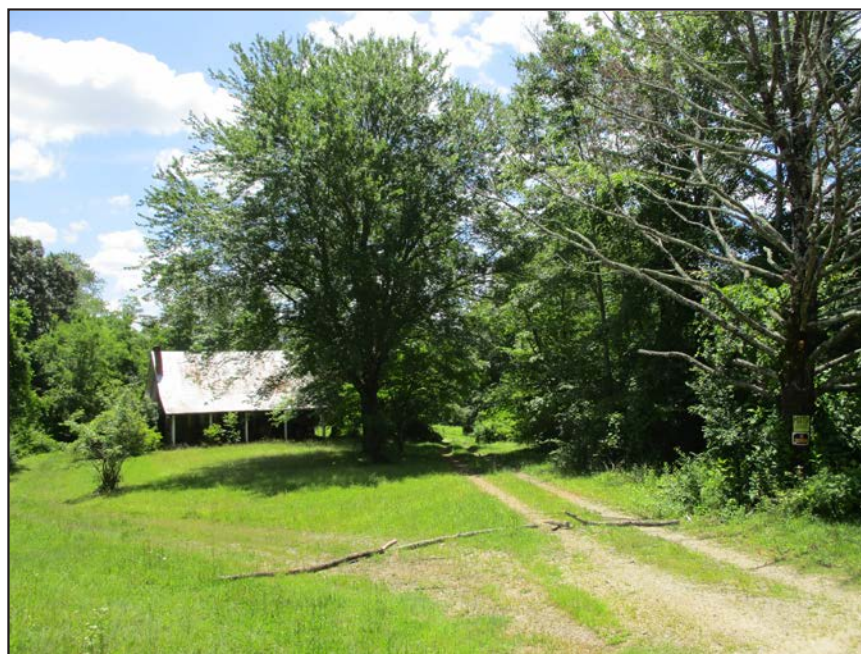
Photograph 2: Façade (northwest elevation) and driveway of J.M. Orders House.; looking southeast. (2017)
