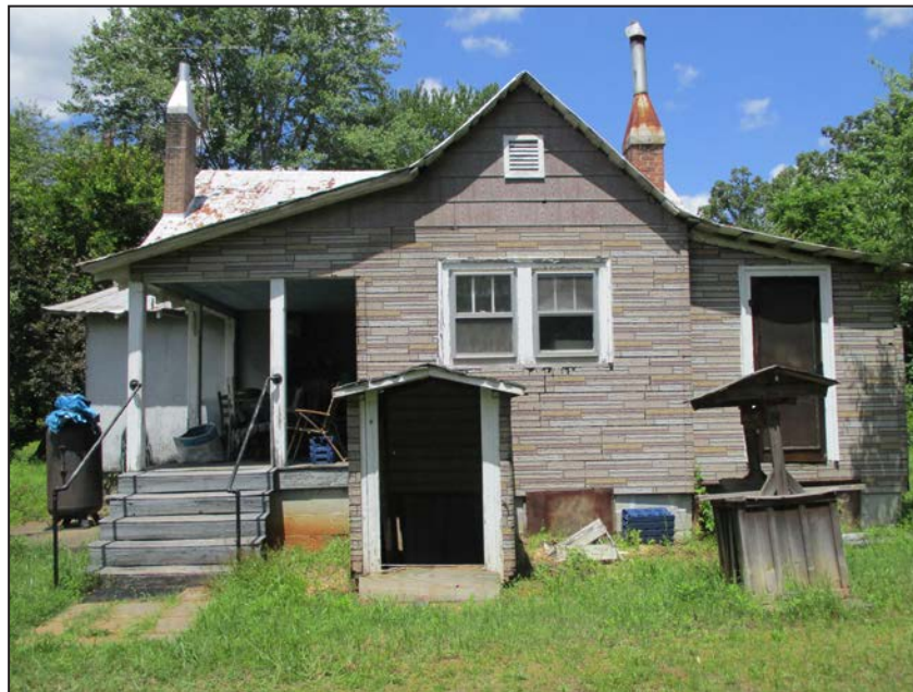
Photograph 7: View of rear (southeast) elevation of J.M. Orders House.; looking northwest. (2017)
