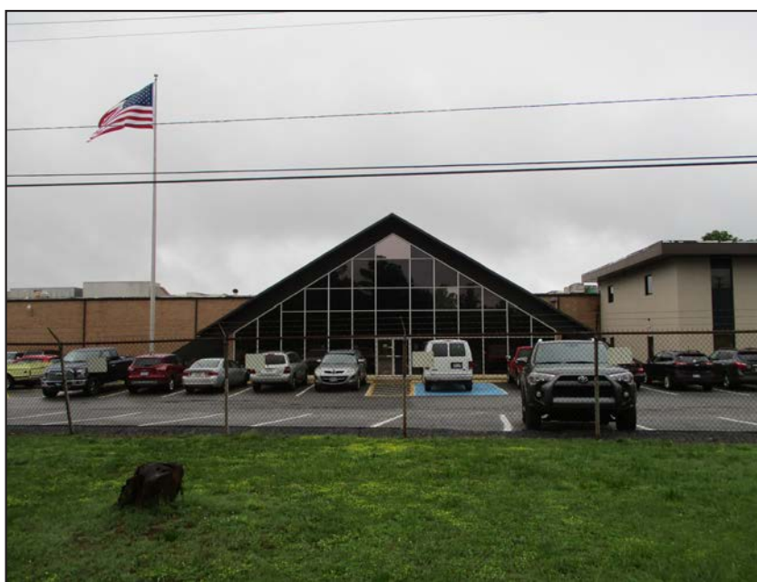
Photograph 15: View of façade and A-Frame entrance bay of Catawba Complex; looking north. (2017)
