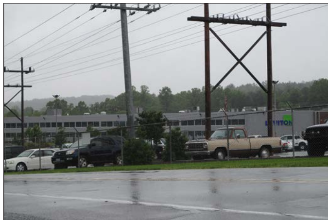
Photograph 16: Leviton Manufacturing Company Industrial Building. (2017)
