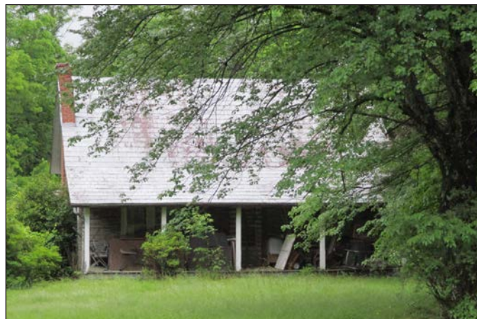
Photograph 1: Façade (northwest elevation) of J.M. Orders House; looking southeast. (2017)
